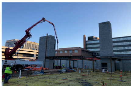
Steel Erection & Concrete Slab:
