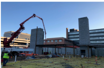
Steel Erection & Concrete Slab:
