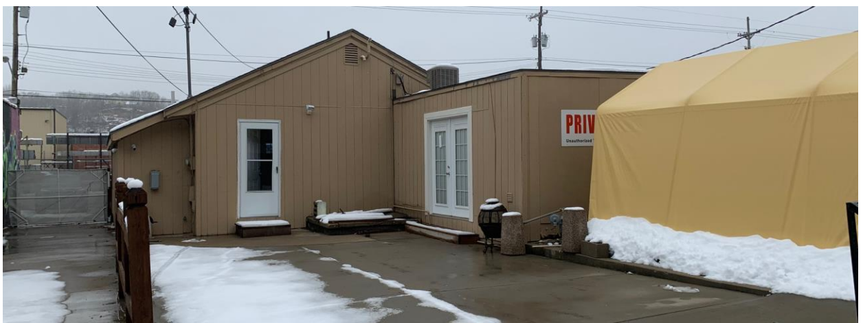
Figure 6. Photograph of the north façade of 1127 Southwest Boulevard (provided by the applicant).
