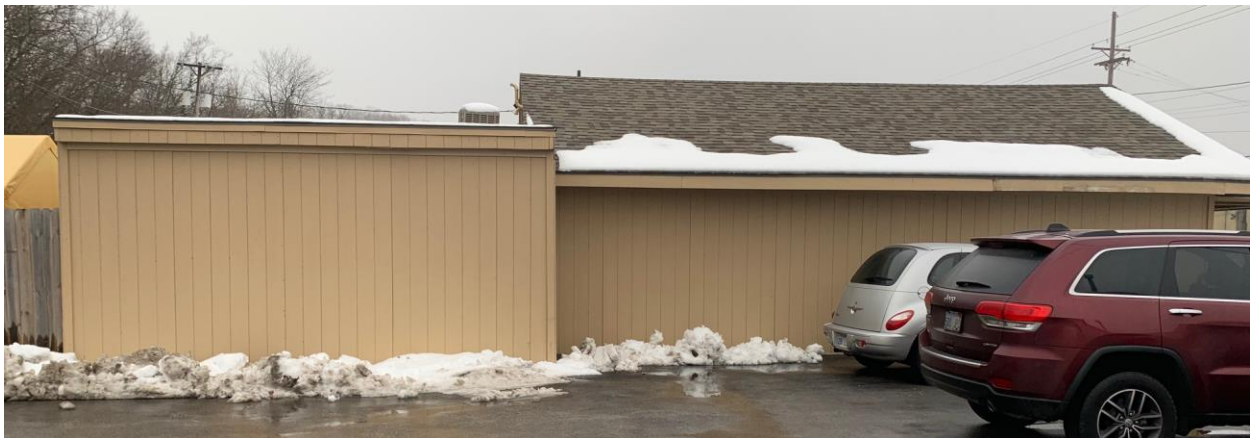
Figure 5. Photograph of the east façade of 1127 Southwest Boulevard (provided by the applicant).
