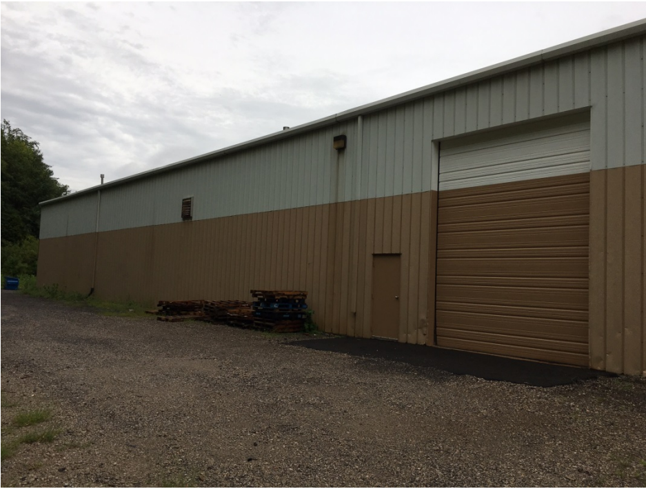
Northeast end of building (looking south)
