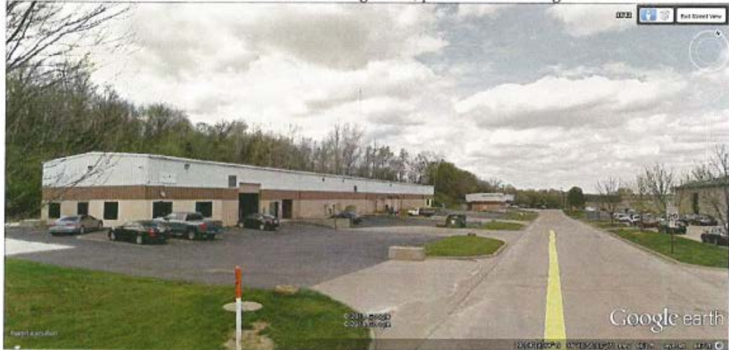
Buried gas line identified in the foreground center.
