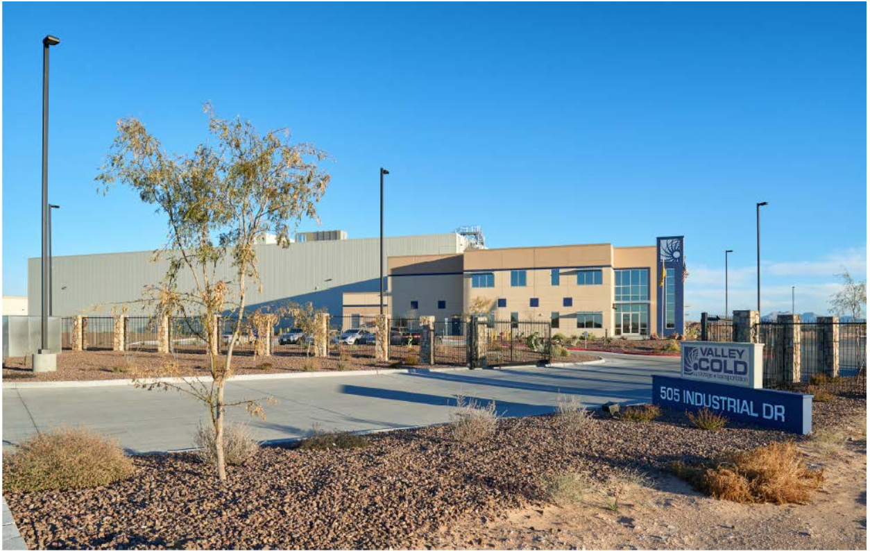
Elevation showing combination of concrete wall panels at the main office and insulated metal panels at the refrigerated storage components.
