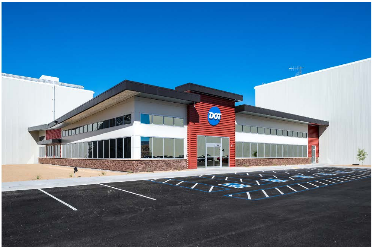
Elevation showing combination of architectural wall panels at the main office and insulated metal panels at the refrigerated storage components.
