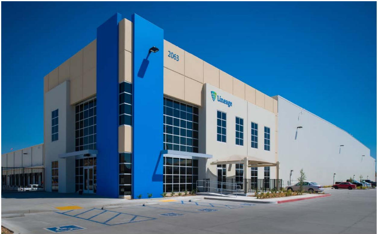
Elevation showing combination of concrete wall panels at the main office and insulated metal panels at the refrigerated storage components.
