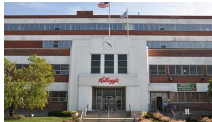
Kellogg's facility located in the Fairfax Industrial District
