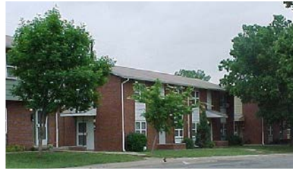
Juniper Gardens public housing complex
