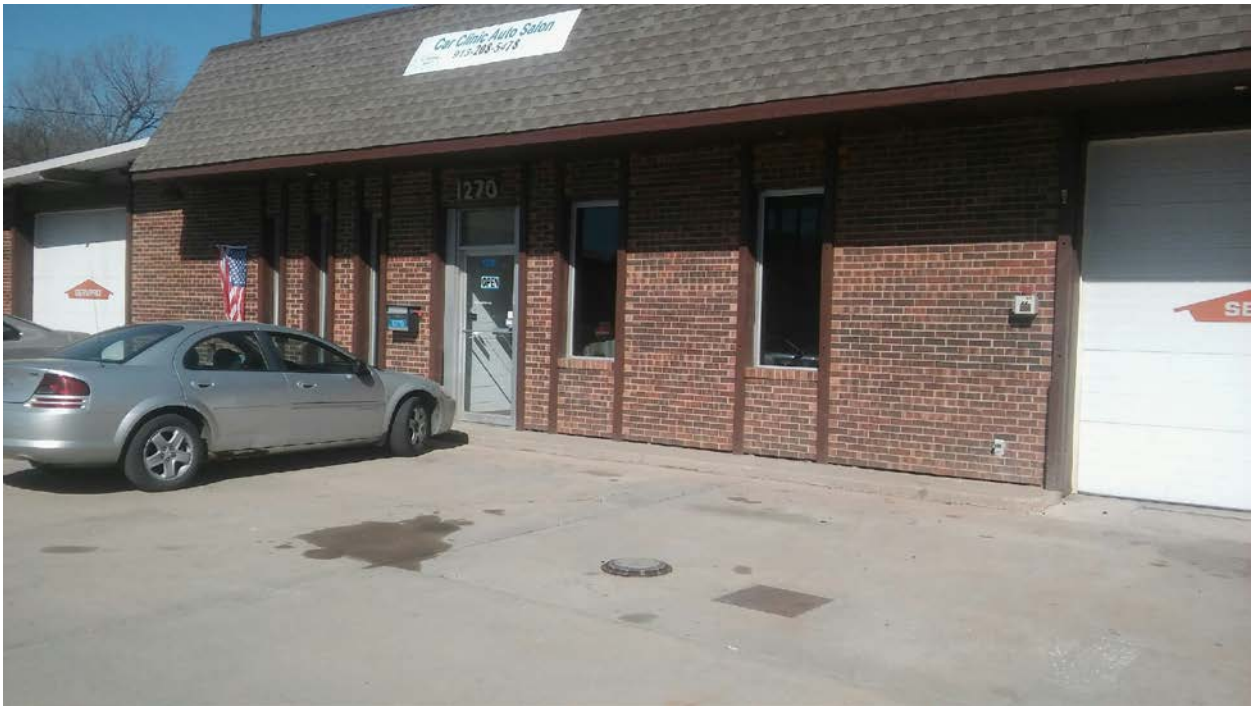
Figure 2. Photograph of 1270 Southwest Boulevard looking north (provided by the applicant).
