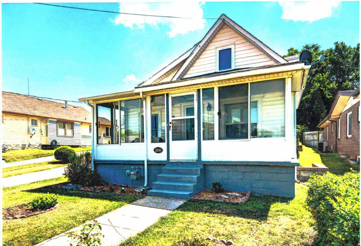
Figure 4. Photograph of 3841 Lloyd Street (provided by the applicant).
