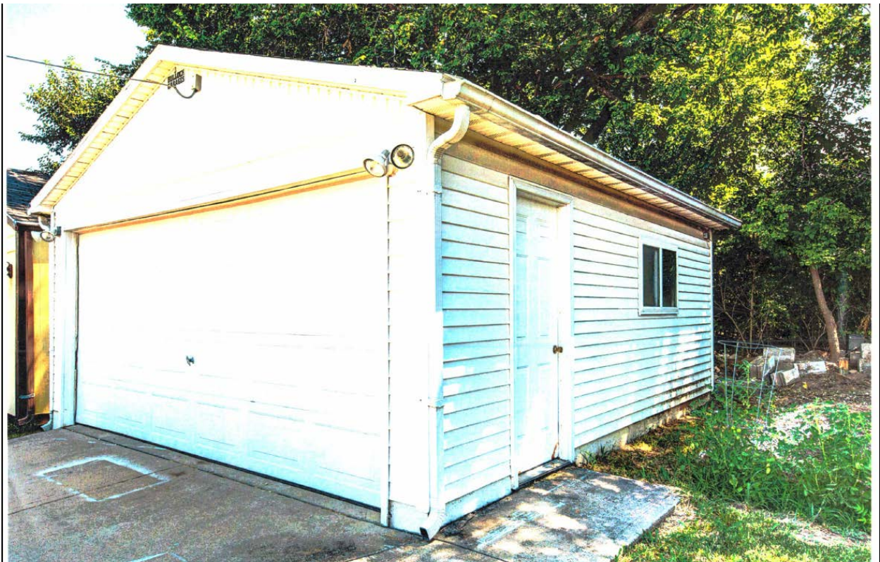
Figure 11. Photograph of the two-car garage at 3841 Lloyd Street (provided by the applicant).
