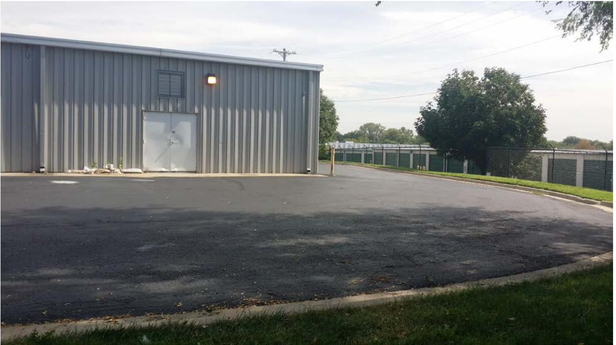
Figure 4. Photograph of 4439 Shawnee Drive looking southeast (provided by the applicant).
