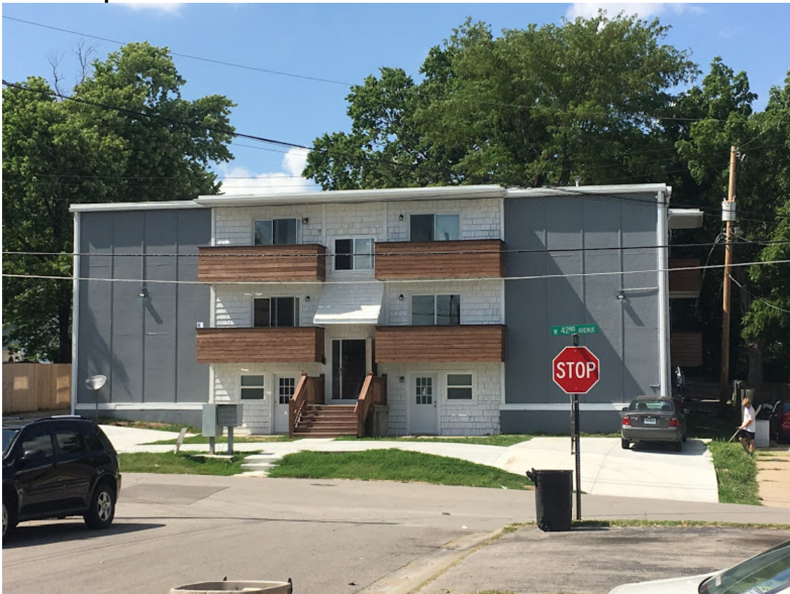
Front of building
