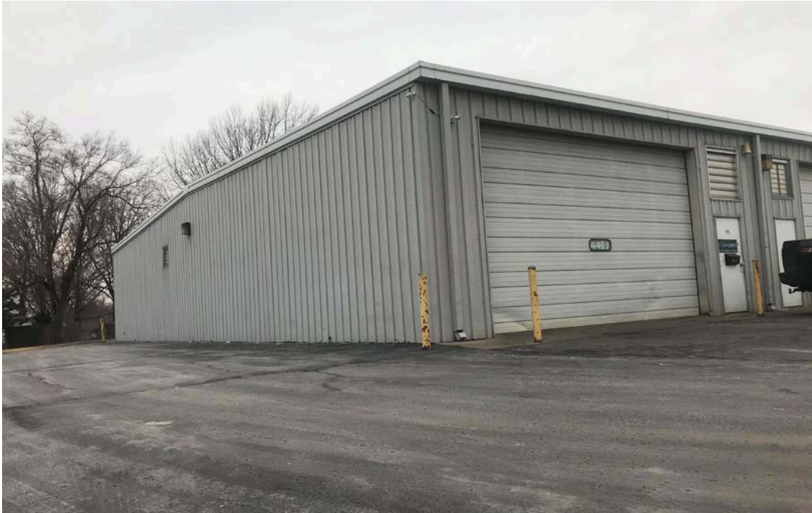
Figure 3. A 2018 photograph of XM Automotive tenant space (provided by the applicant).
