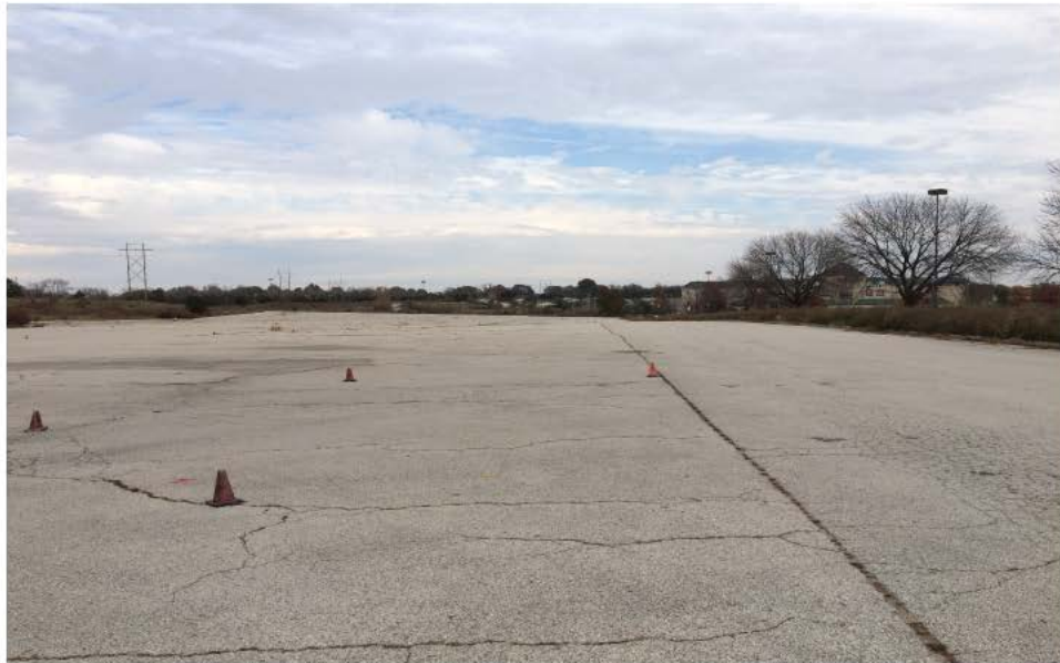
#4) Looking North from South end of West Parking Lot.
