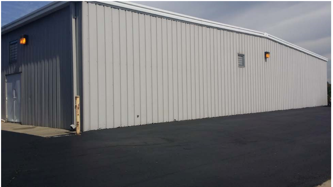
Figure 5. Photograph of 4439 Shawnee Drive looking northeast (provided by the applicant).
