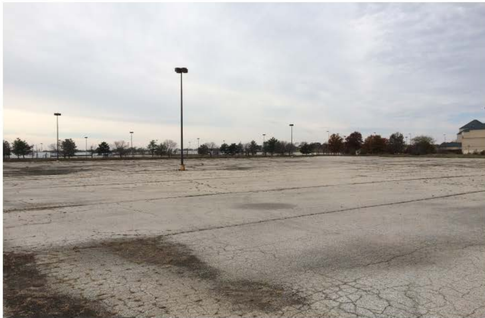
#6) Looking South from North End of Parking Lot East of Dog Track Building.
