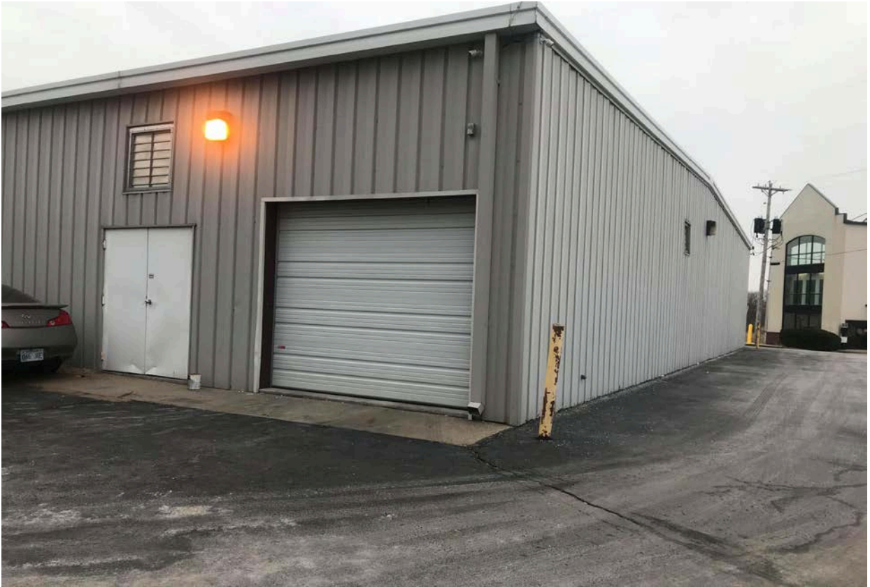
Figure 2. A 2018 photograph of XM Automotive tenant space (provided by the applicant).
