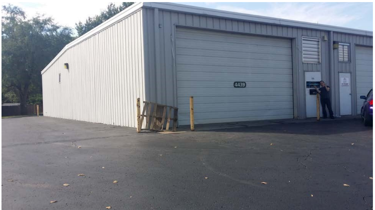
Figure 7. Photograph of 4439 Shawnee Drive looking northwest (provided by the applicant).
