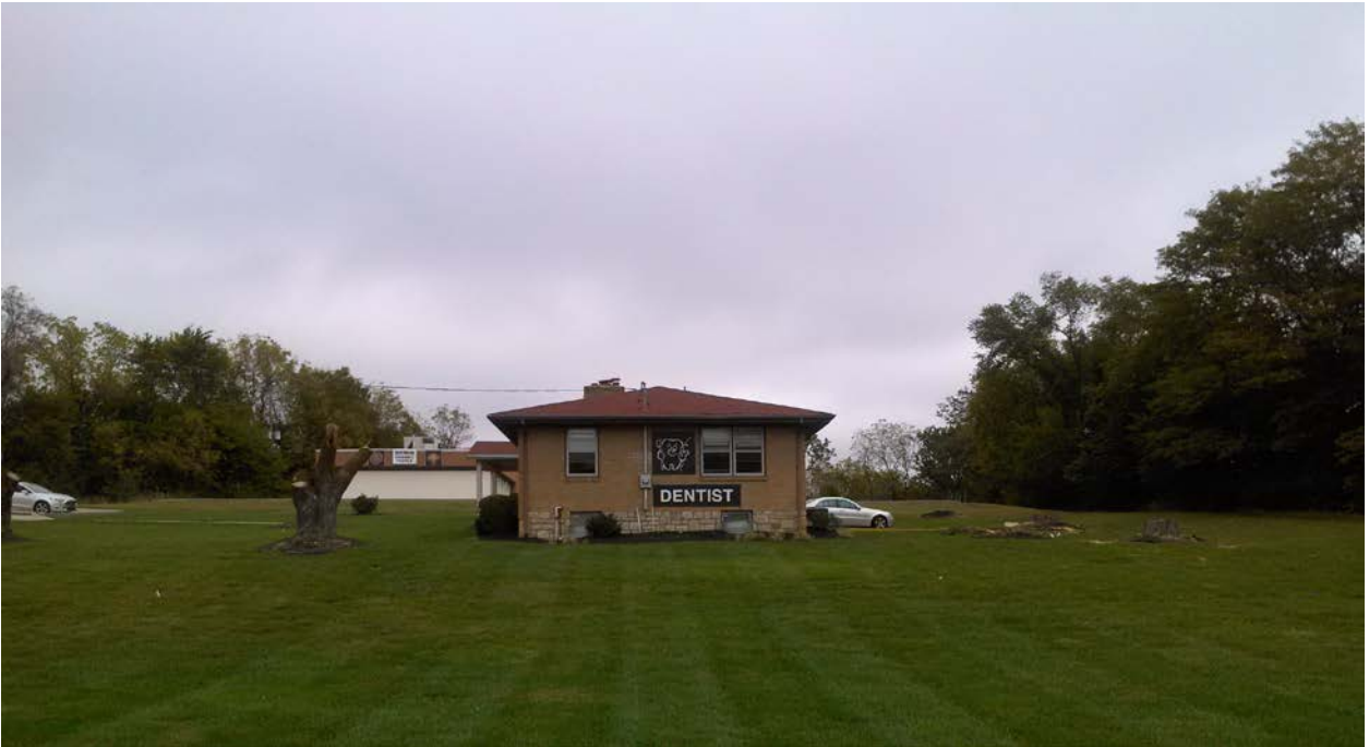
Figure 1. Photograph of existing building at 6708 State Avenue facing south (provided by the applicant).
