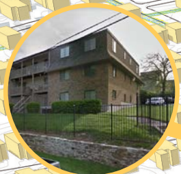
Malvern Hill Apartments
