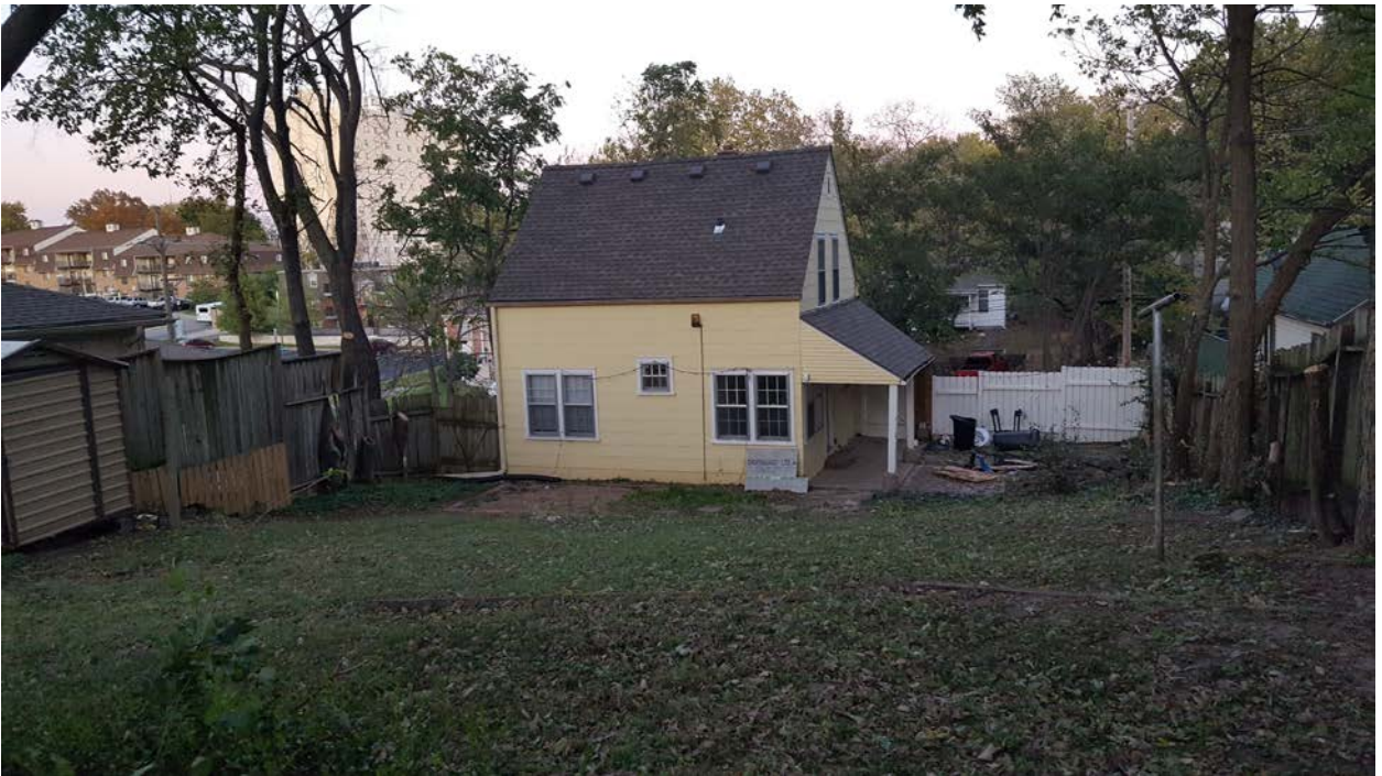
Figure 4. Photograph of rear yard of 3910 Springfield Street (provided by the applicant).
