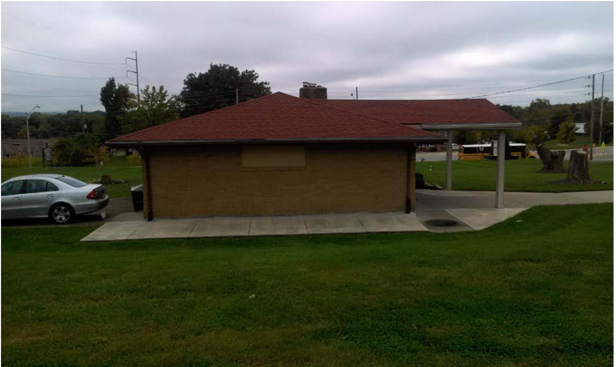
Figure 3. Photograph of existing building at 6708 State Avenue, facing north (provided by the applicant).
