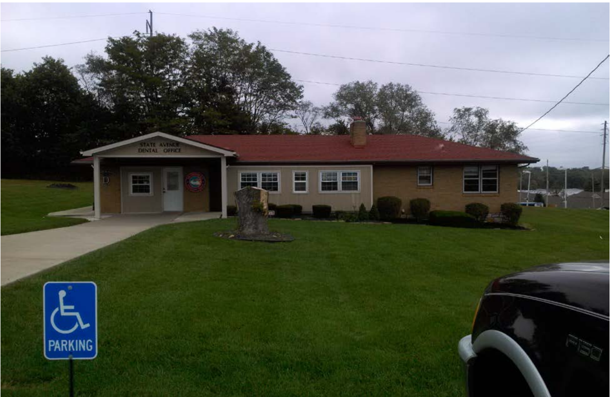
Figure 2. Photograph of existing building at 6708 State Avenue, facing west (provided by the applicant).
