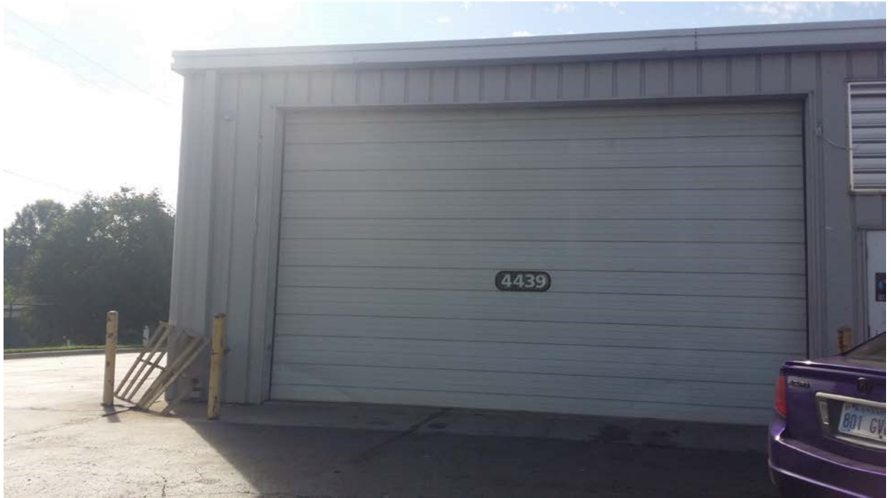
Figure 6. Photograph of 4439 Shawnee Drive looking west (provided by the applicant).
