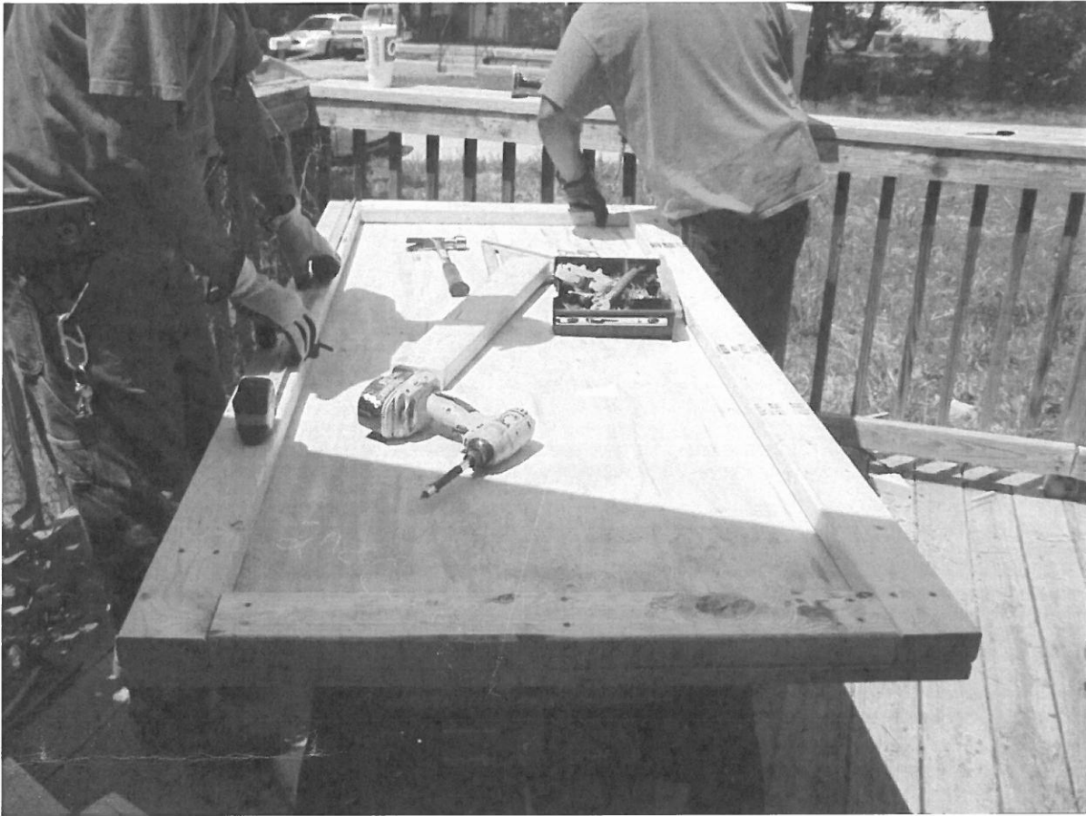
Framed door 2 x 4 and \frac{3}{4} plywood
