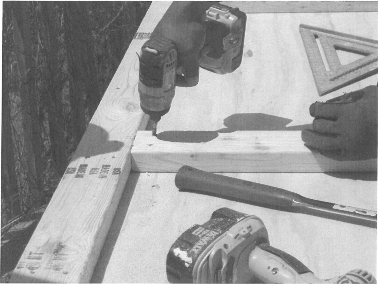
Framed 2 x 4 and three quarter plywood with middle brace
