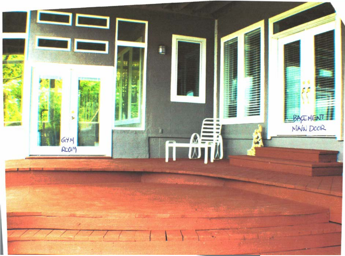
BASEMENT MAIN DOOR & GYM ROOM/STORAGE
