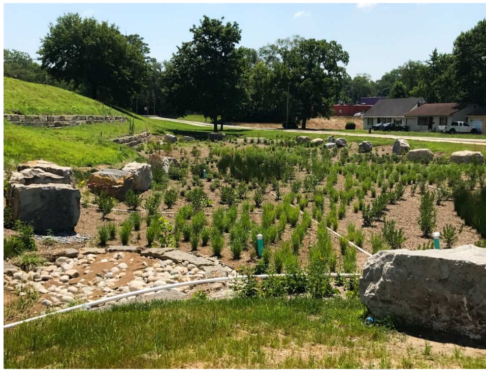
Figure 5 Example of a Bioretention Facility Integrated into a Low Area of a Park (Arleta Park, Kansas City, MO)
