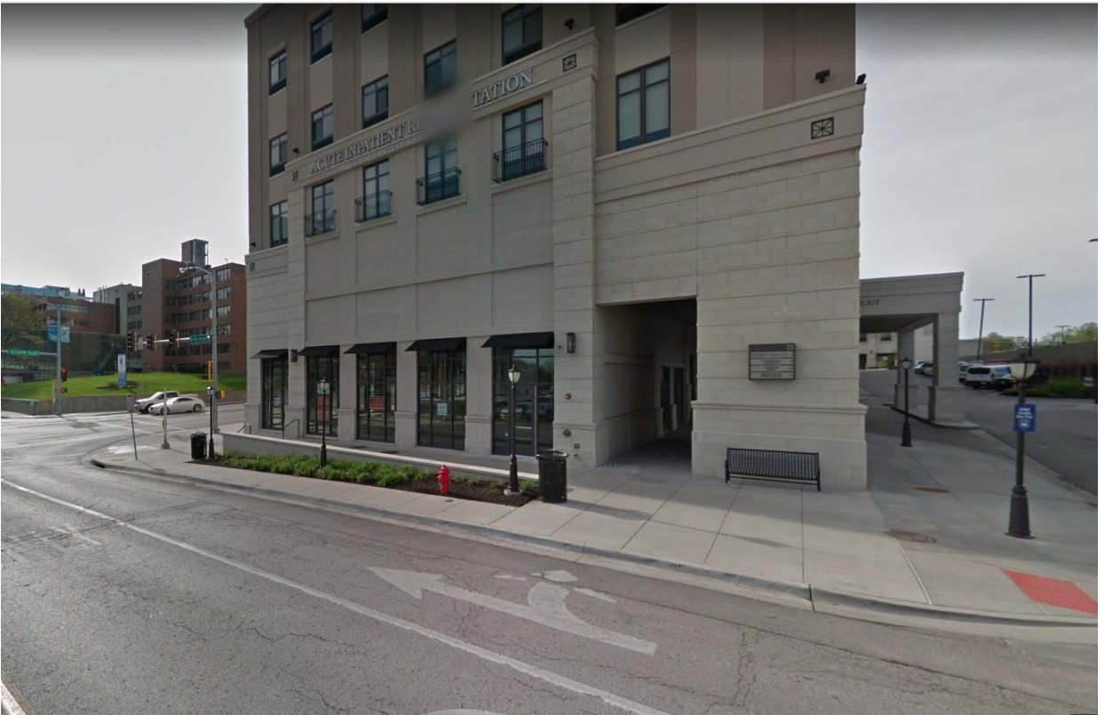
Figure 2. Site photograph of 3900 Rainbow Boulevard (provided by Google Street View).
