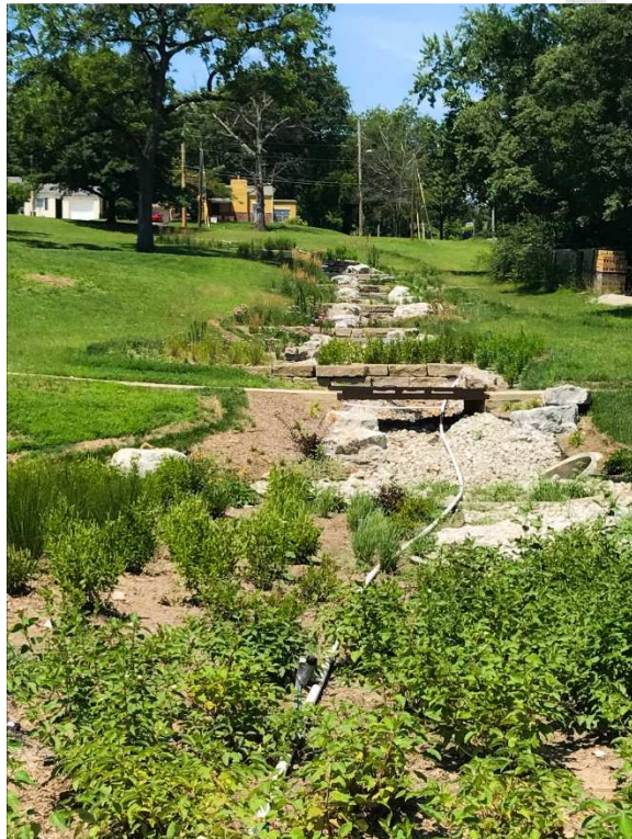
Figure 4 Example of Dry Creek Bed for Stormwater Conveyance on Steep Slopes (Arleta Park, Kansas City, MO)
