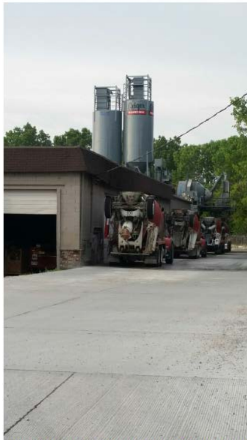
Photo 10- One way access drive and staging lane for wet batch plant.
