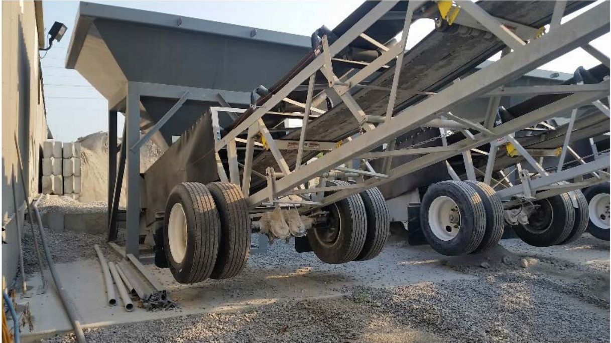
Photo 5-concrete under aggregate loading hoppers.
