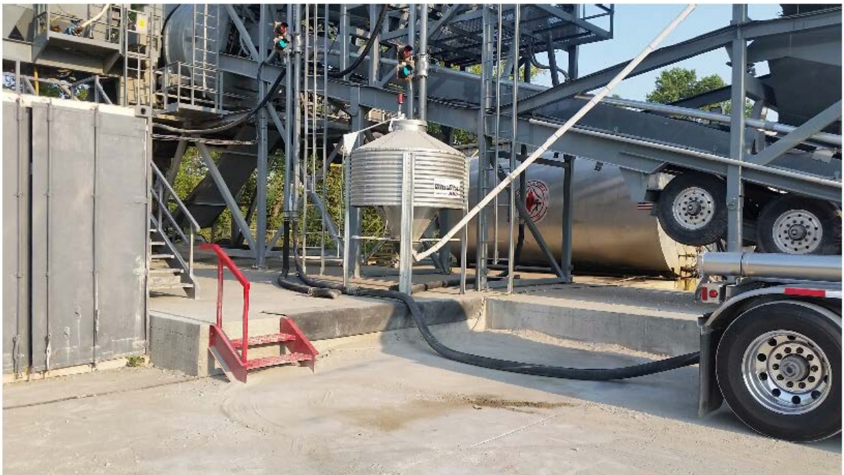
Photo 4-concrete slab under base of plant.
