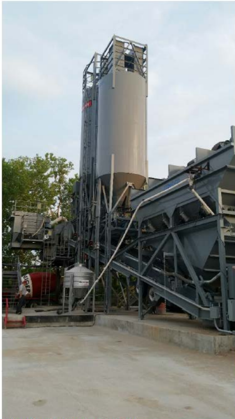
Photo 11-Concrete slab under wet batch plant
