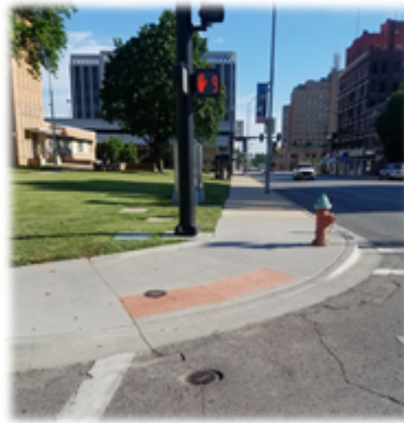
New Pedestrian Ramp/Signal
