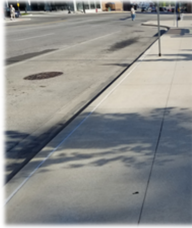
New Curb and Sidewalk
