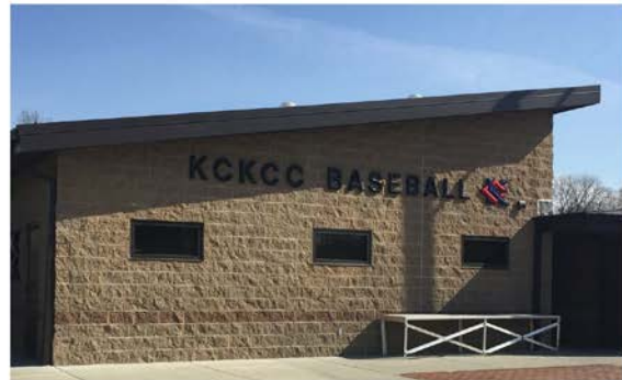
Existing Adjacent Building
