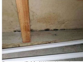
Basement (Behind Water Heater)
