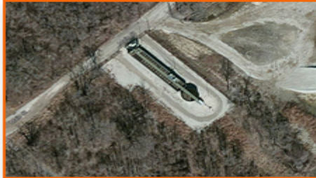
Existing Package Plant
