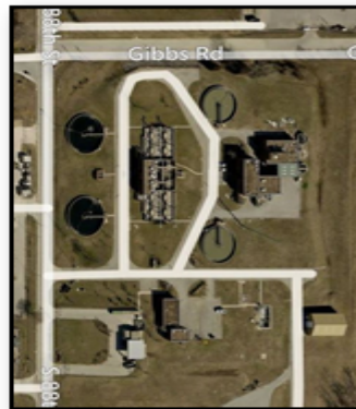
Permanent Treatment Plant
