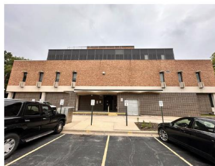
View from the South
