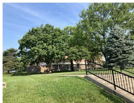
View from the Southeast
