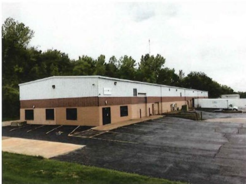
View of the south end of building and property, (looking northwest)
