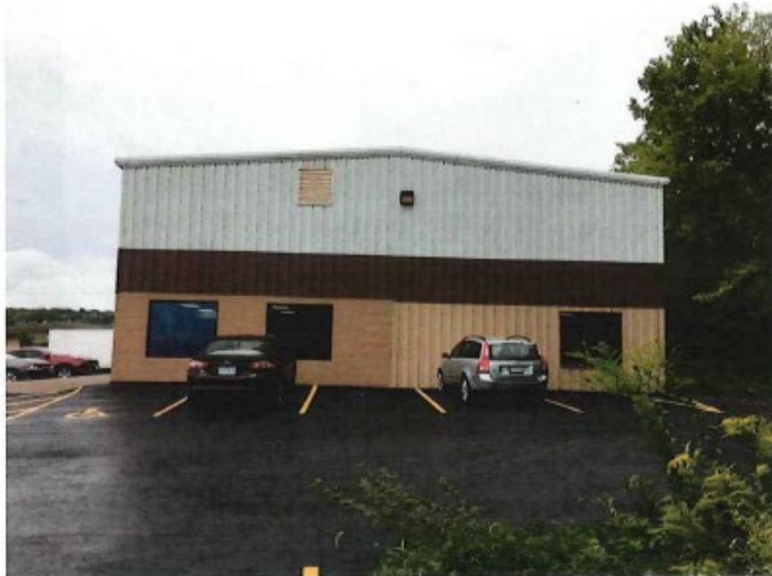
Northend of building (looking south)
