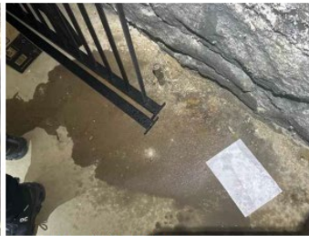
Basement below shower
