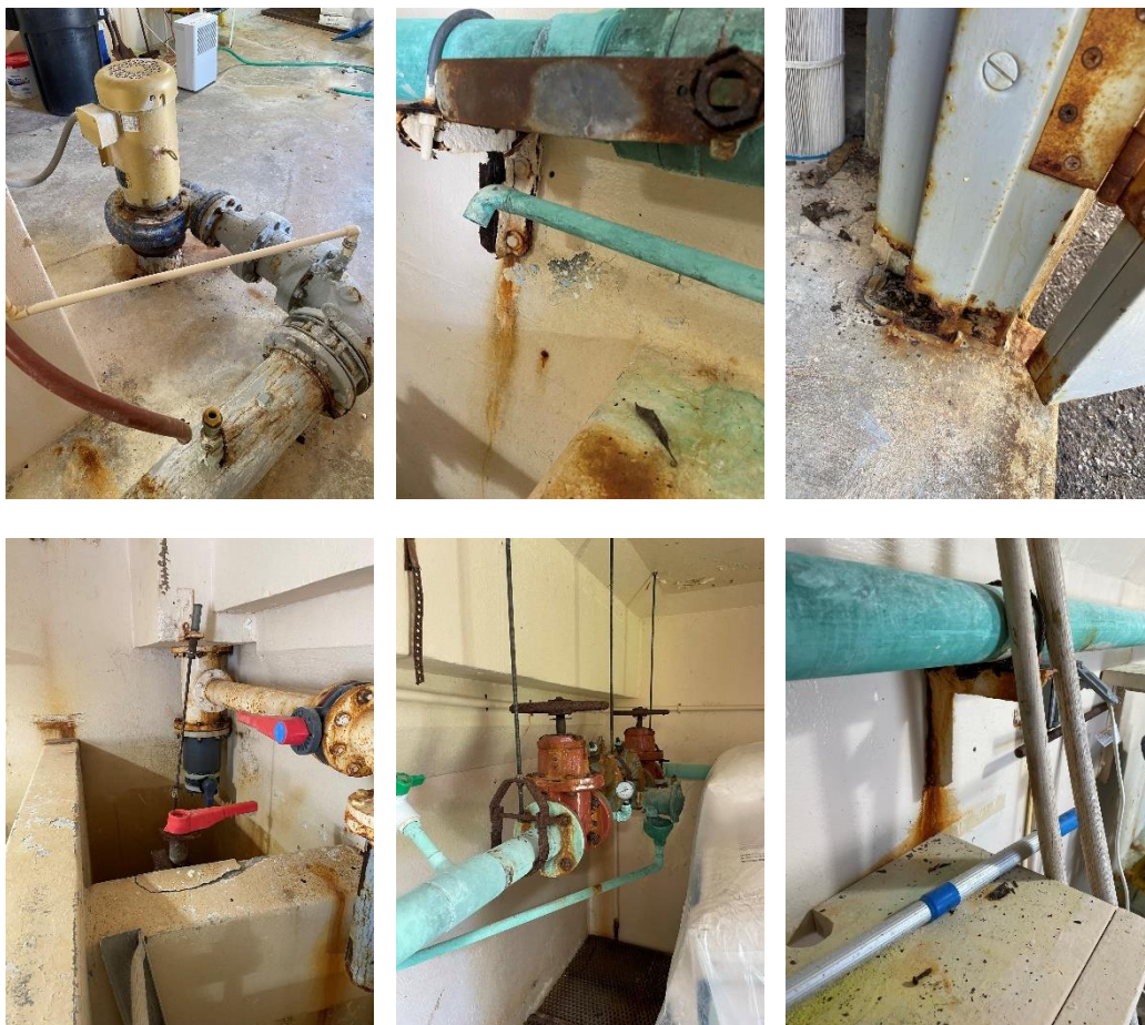
Corroded Components
