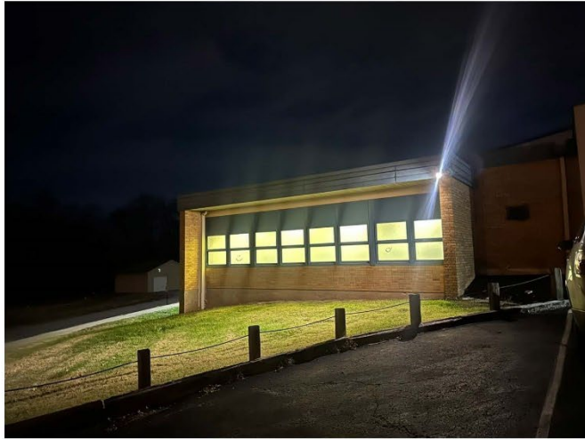
West end of building on south, looking to the north-west of site.
