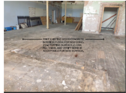
1 INTERIOR CONCRETE RESURFACE NO SCALE
