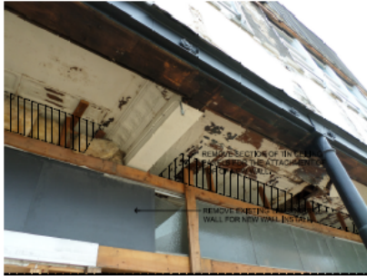
1 EXTERIOR CEILING DEMOLITION NO SCALE
