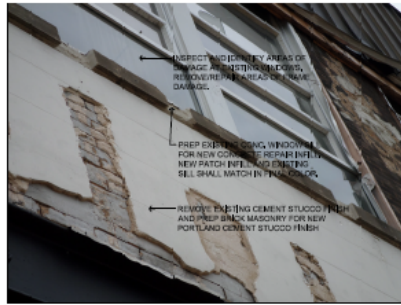
1 EXTERIOR WALL SURFACE DEMOLITION NO SCALE
