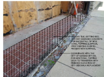
1 EXTERIOR CONC. DEMOLITION NO SCALE
