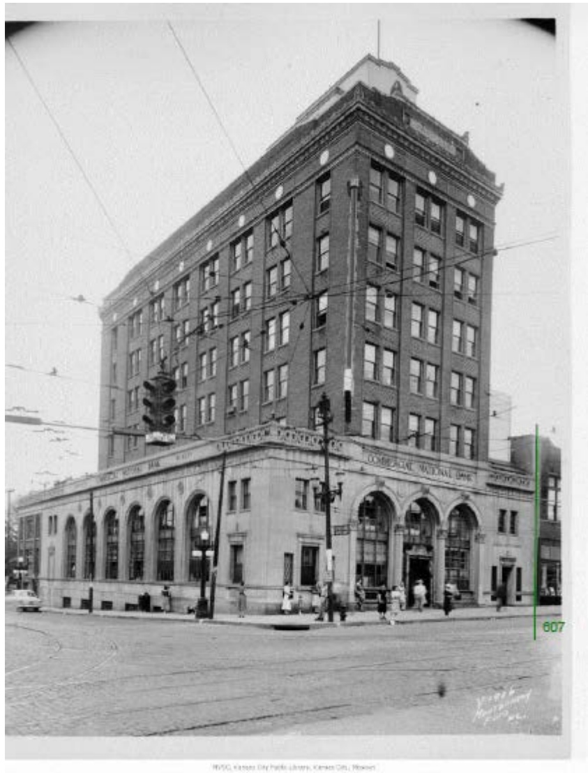
W.C. Clegg Building, Kansas City Public Library, Kansas City, Missouri
