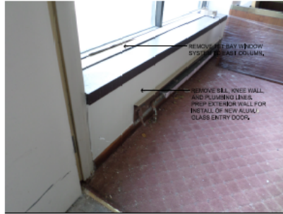
1 DEMOLITION @ NEW ENTRY(607A-EAST) NO SCALE
